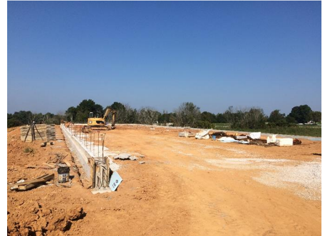
Perimeter Foundations (A & B)
