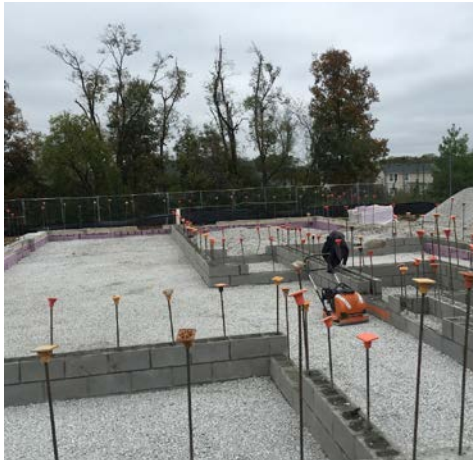
Gravel Under Slab
