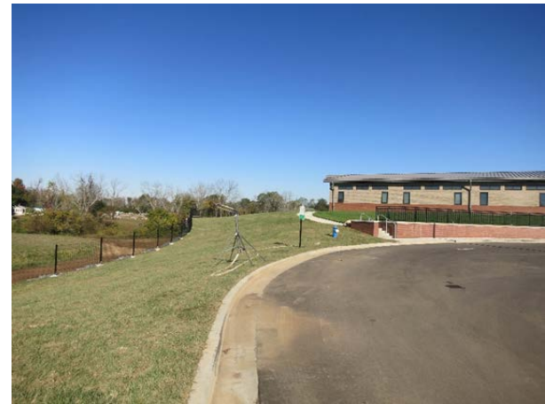
Sod Installation at Front
