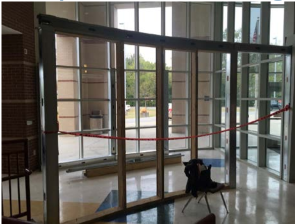
Temp Curtainwall Framing
