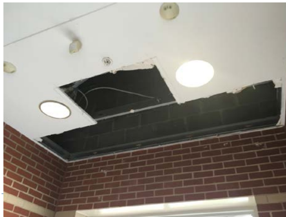
Ceiling Demo for New HVAC Duct
