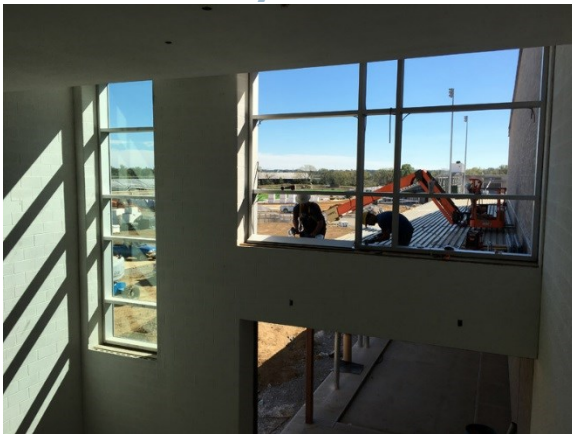
South Entry Curtain Wall
