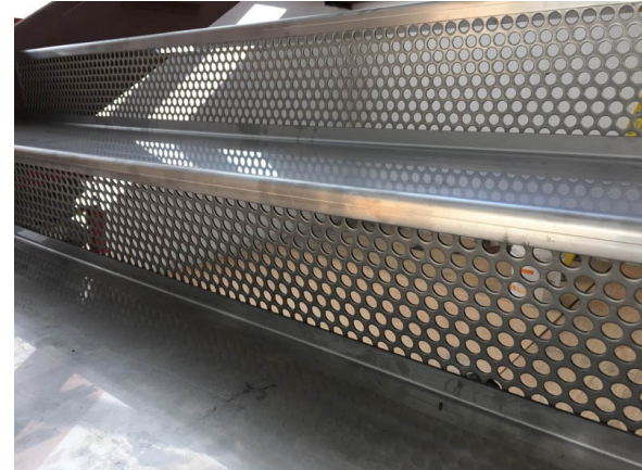
Stair – Stainless Steel Risers
