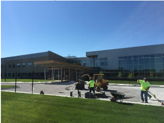
North Entry – Permeable Pavers
