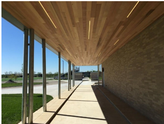
South Entry Canopy
