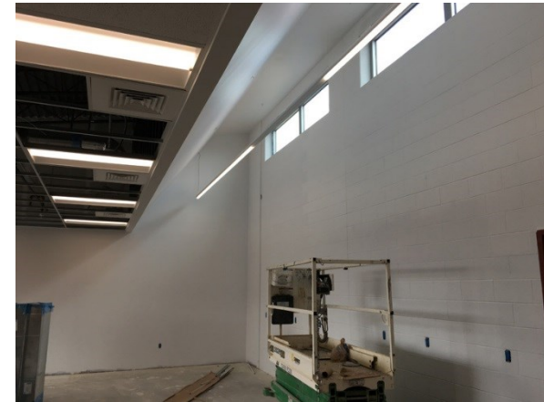
Art Room Clerestory
