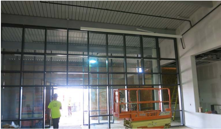
Front Entry – Curtain Wall
