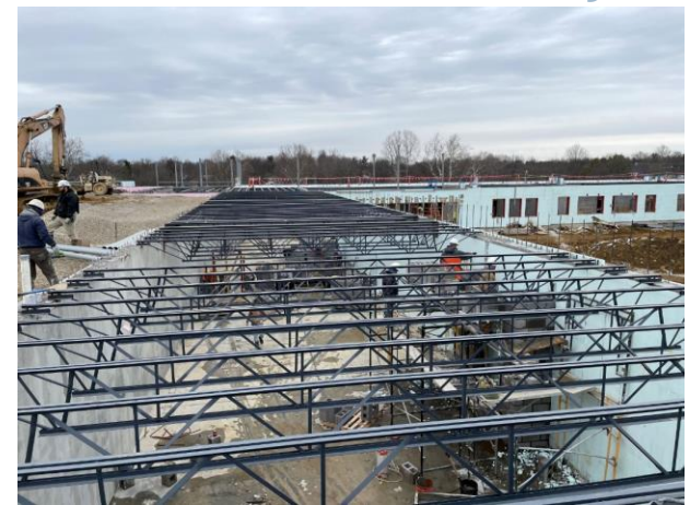
Area D – Lower Level Steel Joists
