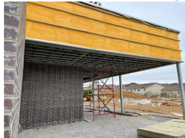
Fieldhouse – Soffit Framing
