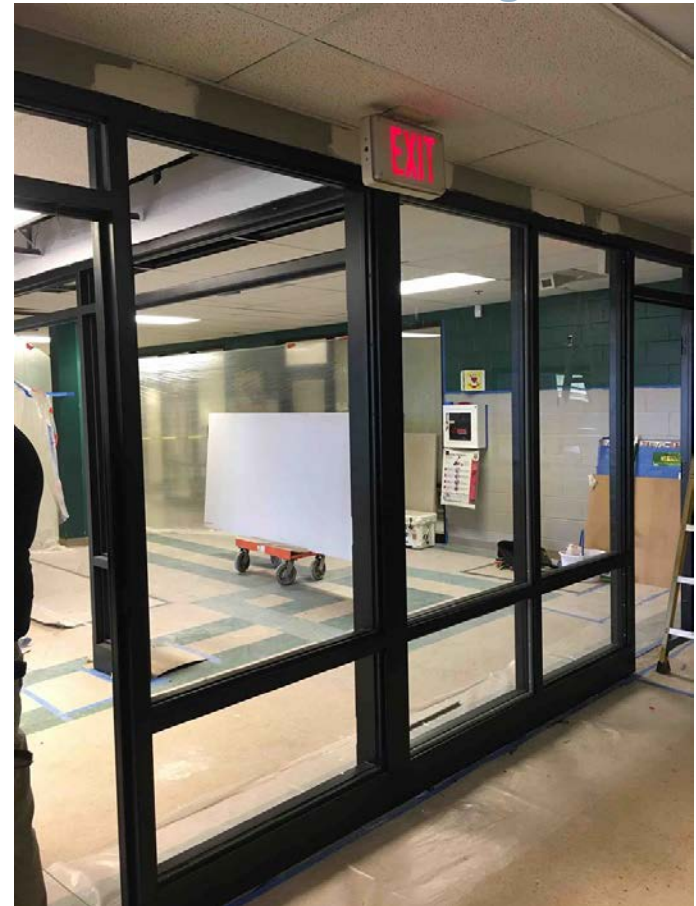
New Door Frame Creating Vestibule
