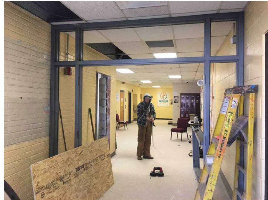
New Hollow Metal Frame
