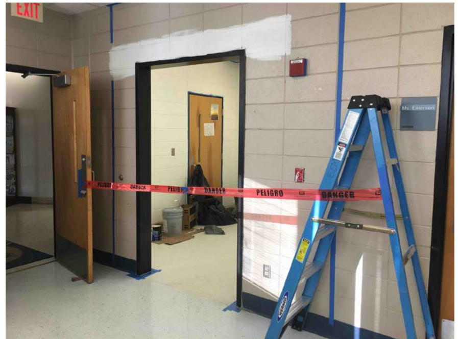
New Wall Opening at Reception
