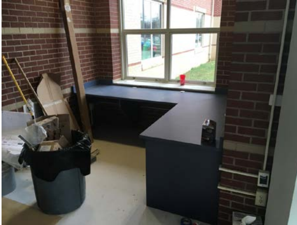
New Secure Vestibule Office
