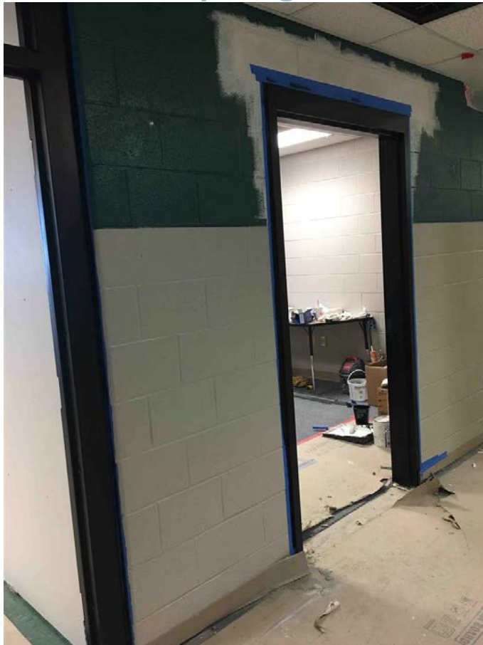
New Door Opening in CMU Wall
