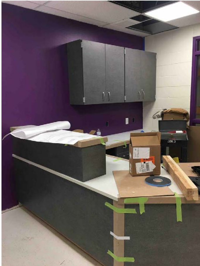
New Reception Casework
