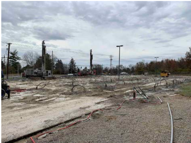
Geothermal Drilling
