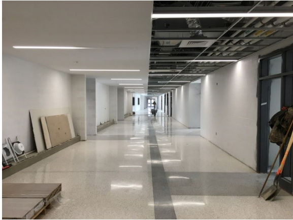
1 st Floor Corridor (Area B)
