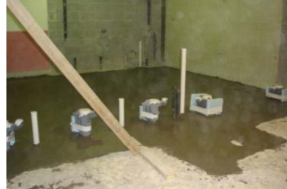
Replacement Slab in Restrooms
