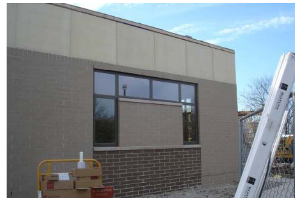
New Addition – Jumbo Brick & Cast Stone Panels
