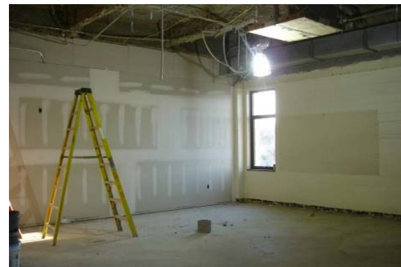
Classroom – New Drywall & Windows
