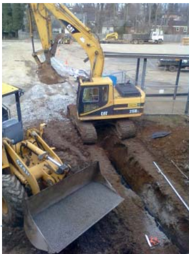
Admin Area Foundations
