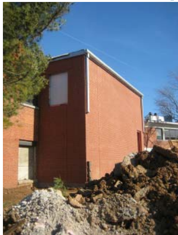
New Exit Stairway
