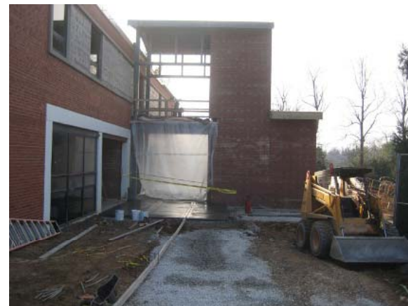
New Elevator Addition
