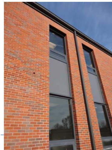
New Window Panels
