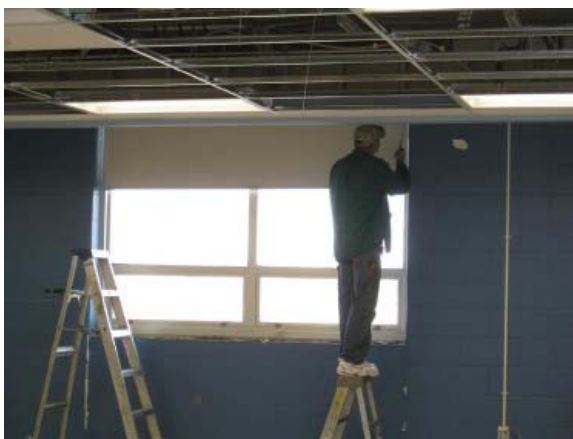
Installation of Window Treatments
