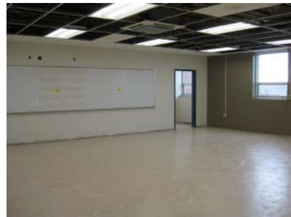
VCT Flooring in Classrooms
