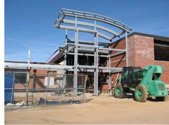
Entry Vestibule Framing
