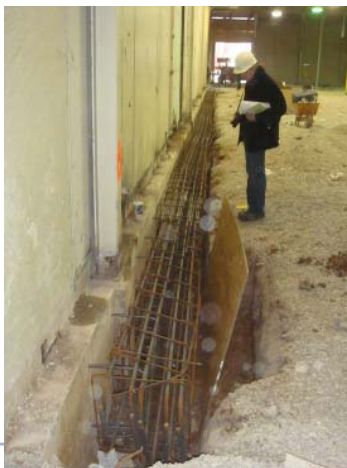
Grade Beam Rebar
