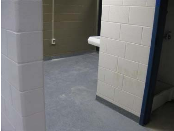
Epoxy Flooring in Restrooms
