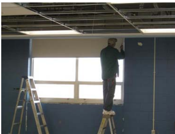
Installation of Window Treatments
