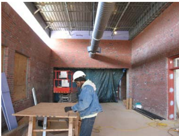
Phase I Lobby
