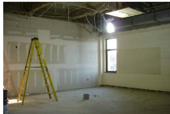
Classroom – New Drywall & Windows
