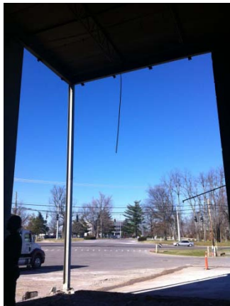
Concrete Panel Demo
