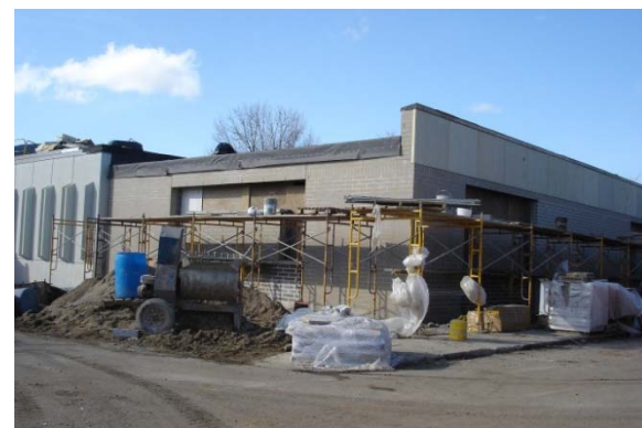
Back & Side of Addition
