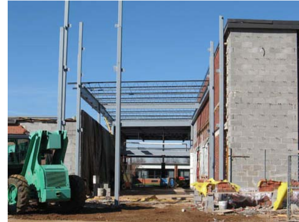
Lobby - Structural Framing
