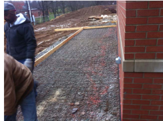
Installation of Concrete Sidewalks
