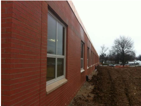
New Classroom Wing
