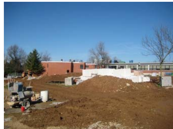
New Mechanical Room Addition
