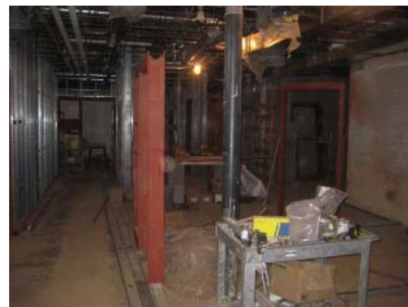
Lower Level Corridor
