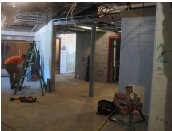
Front Entry Corridor
