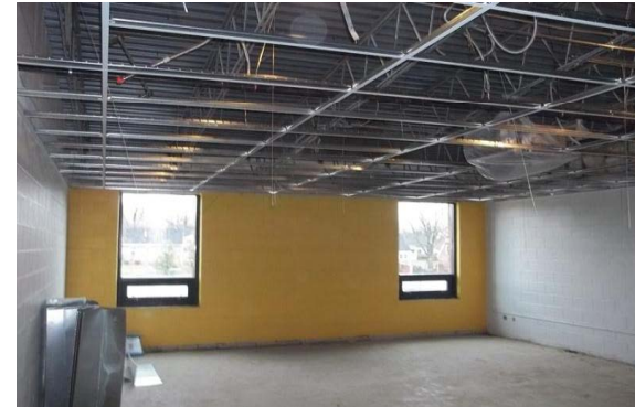
Classroom Ceiling Grid
