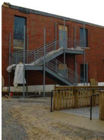
Exterior Temporary Stair
