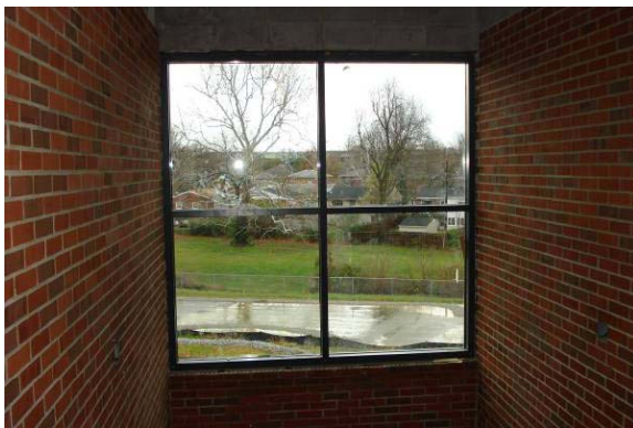
New Windows Installed
