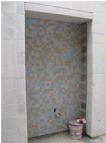
Tile Backsplash in Corridors
