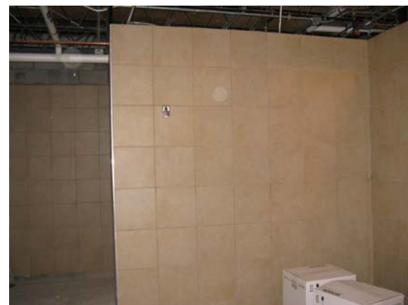
Ceramic Tile Walls in Restrooms
