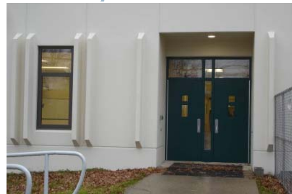
New Entry Doors to 2 nd Floor
