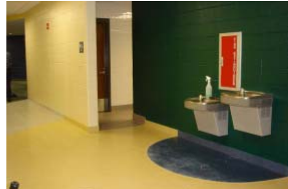
Hallway -- New Terrazzo Floor
