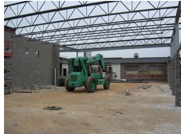
Media Ctr. Steel Erection
