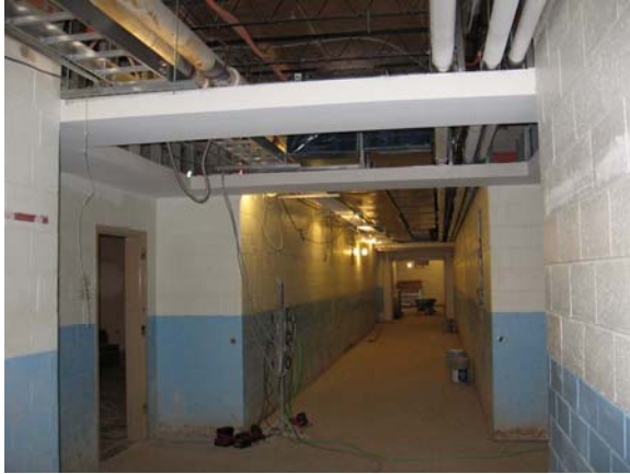
MPE Installation in Corridor
