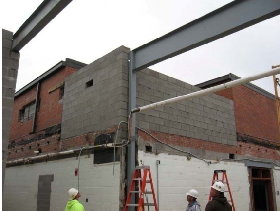
Corridor & Lobby Construction
