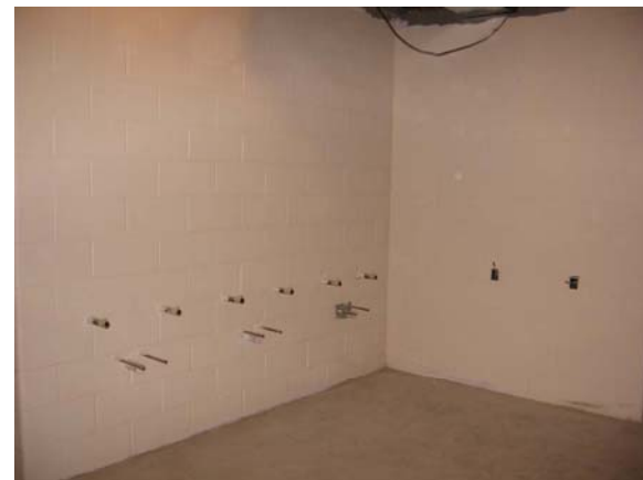
Gang Restroom Rough-ins
