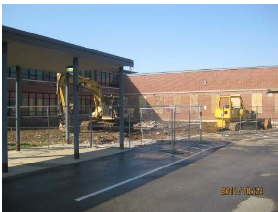
Earthwork – Admin. Area
