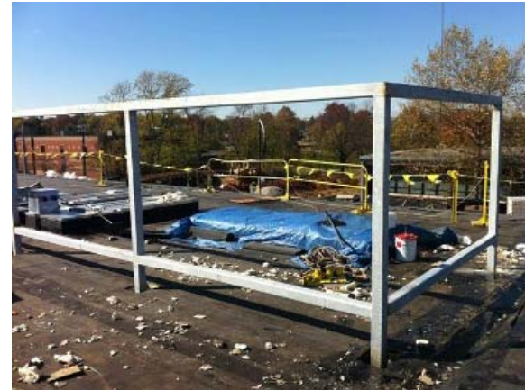
Installation of HVAC Equip.
