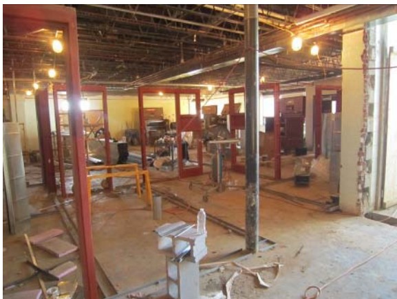
Area A Lower Level
