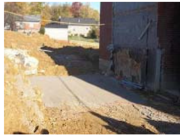
Grade Work at Elevator Pit
