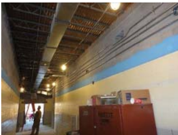
Overhead MEP Rough-ins
