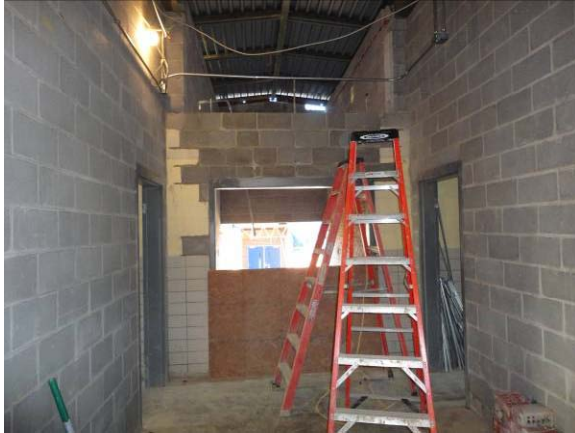
Interior CMU Wall
