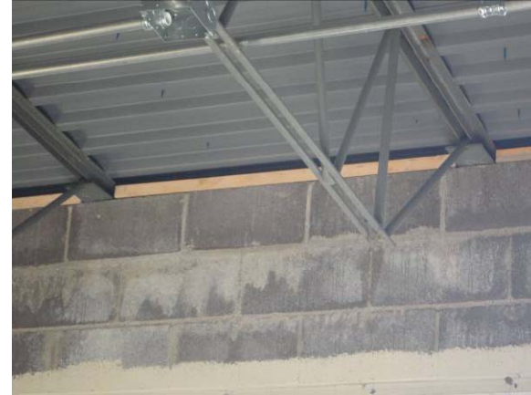
Roof Edge Blocking & Decking
