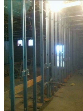
Interior Metal Framing
