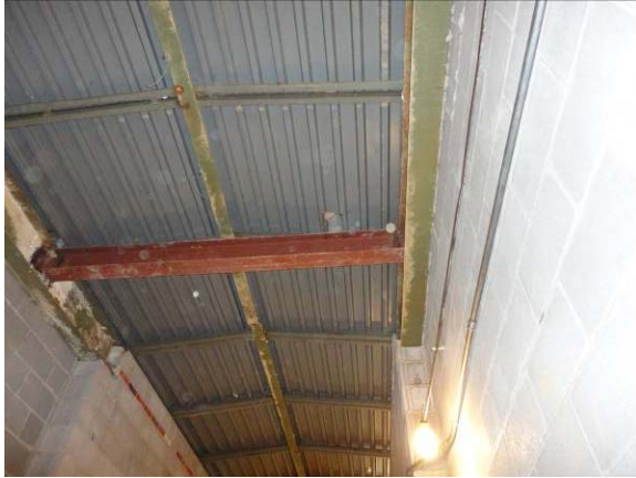
New Steel Work Complete
