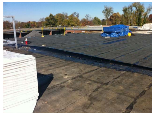
Reroofing of Existing Areas
