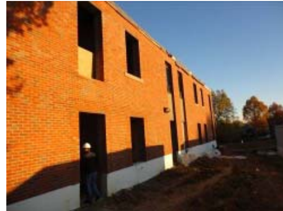
Brick Patched & Washed at New Openings
