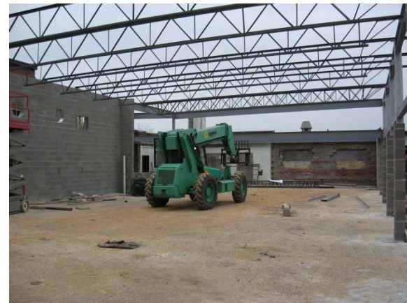
Media Ctr. Steel Erection
