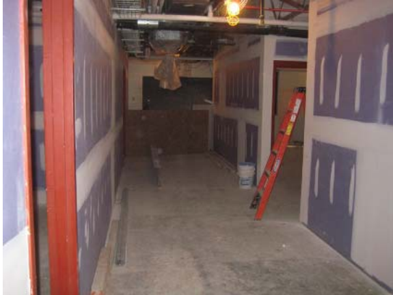
Upper Level Classroom Corridor
