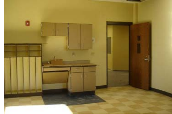
New Casework & Doors
