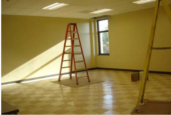
New Flooring & Ceilings
