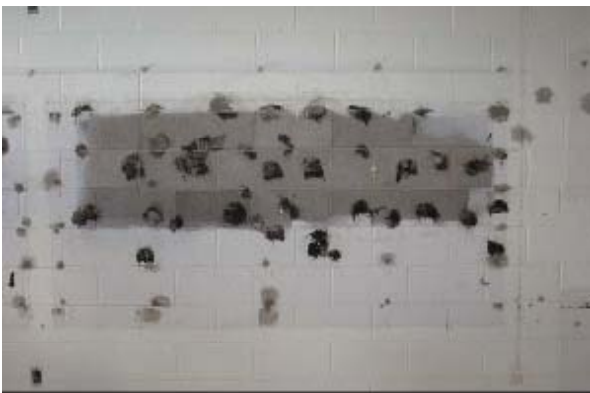
Hazardous Material Abatement
