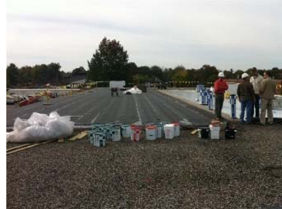
New Roof System
