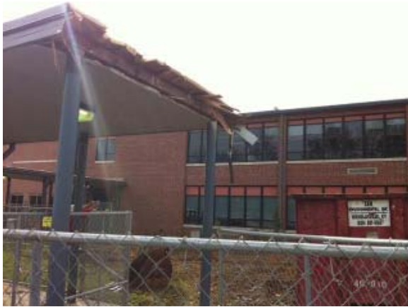
Demo of Existing Canopies
