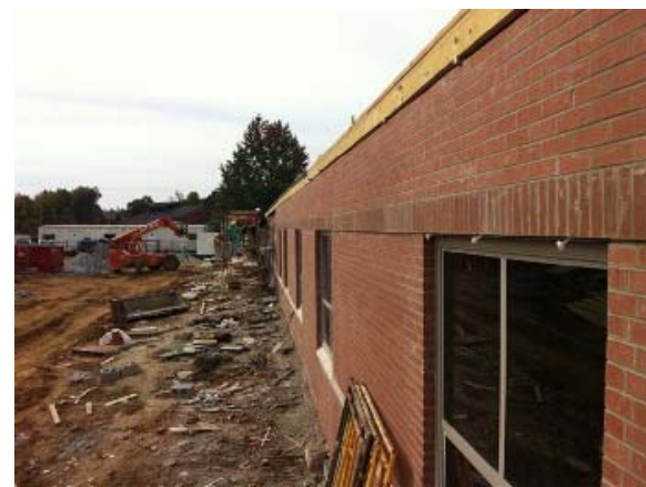
Wood Blocking for Roof Trim
