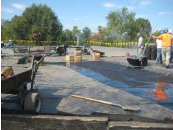
Temporary Roof Installation
