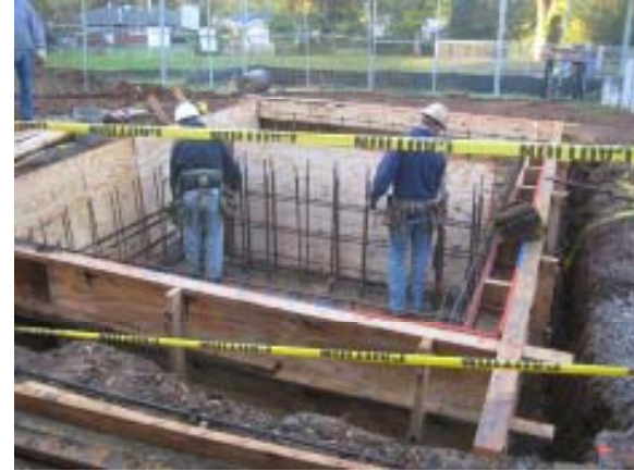
Elevator Foundation & Reinforcement
