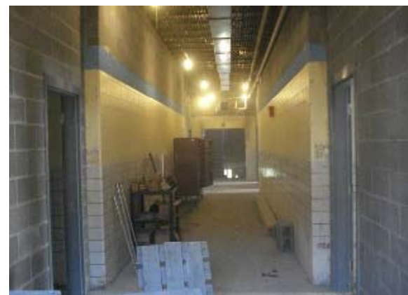
New Interior Corridor & Door Frames
