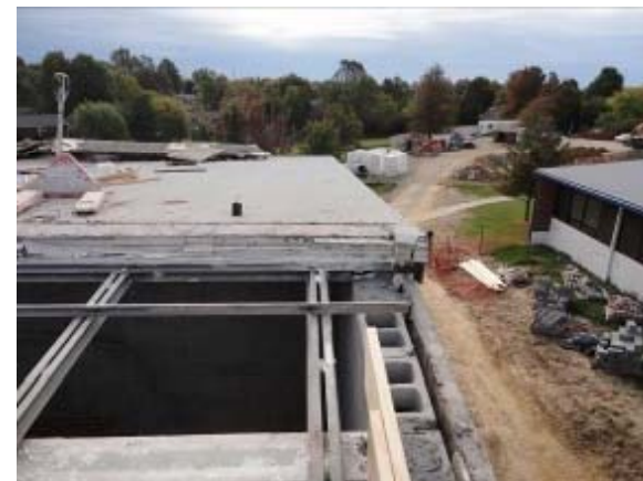
Existing Roof to be Removed
