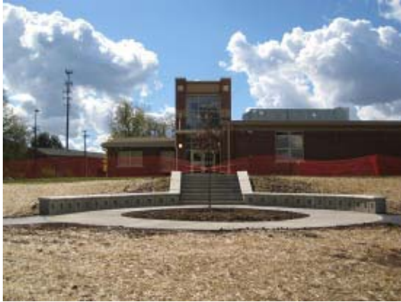
Vestibule & Outdoor Classroom
