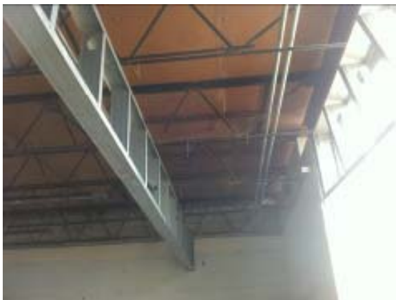
Classroom Metal Soffits
