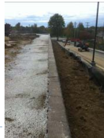
Retaining Wall Complete
