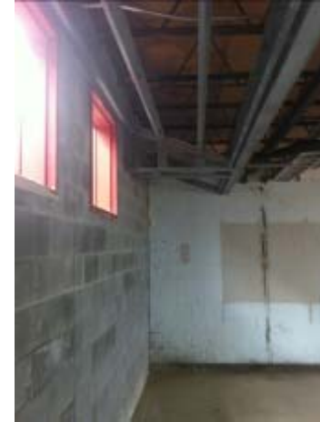
Classroom Metal Soffits
