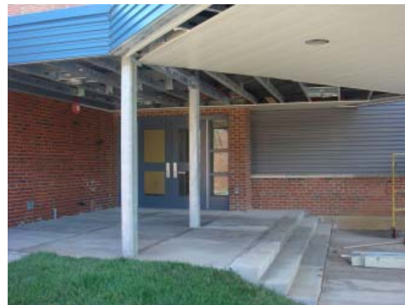
Bus Loop Canopy
