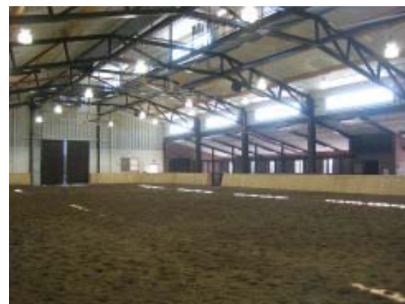
Arena – Riding Surface with Stalls
