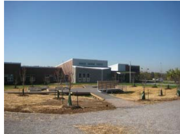
Academic Bldg. – Main Entry
