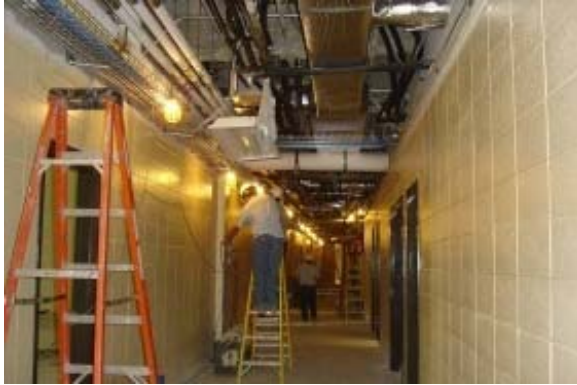
Renovation of Existing Bldg.
