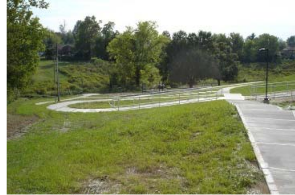
New Ramp & Stairs to Stream
