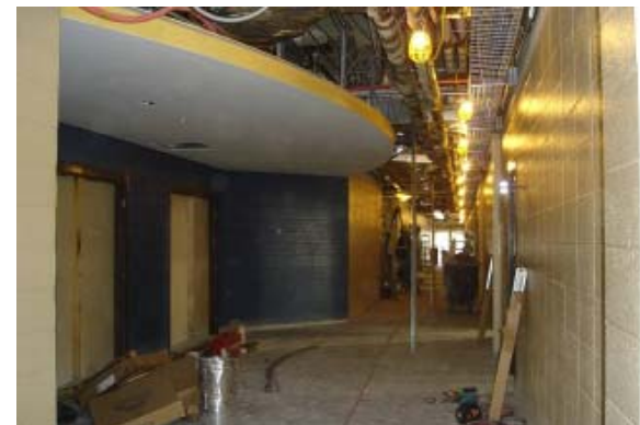
New Soffit – Media Center & Cafe
