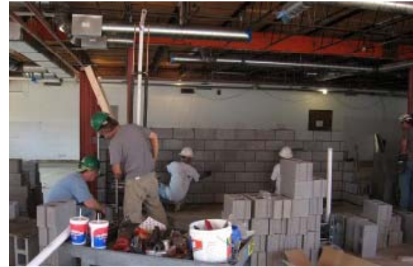
Interior Partition Work
