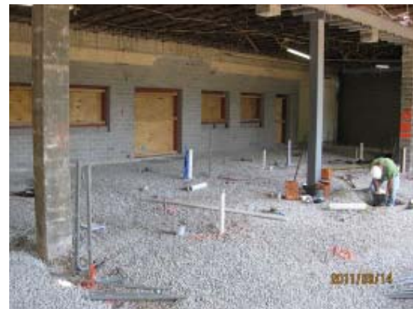
Kitchen – Underground Utilities
