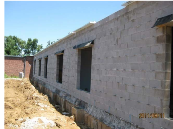
New Block Wall
