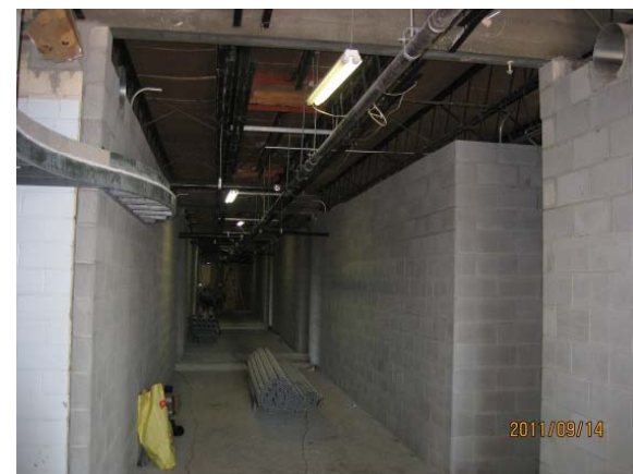
Renovated Classroom Area
