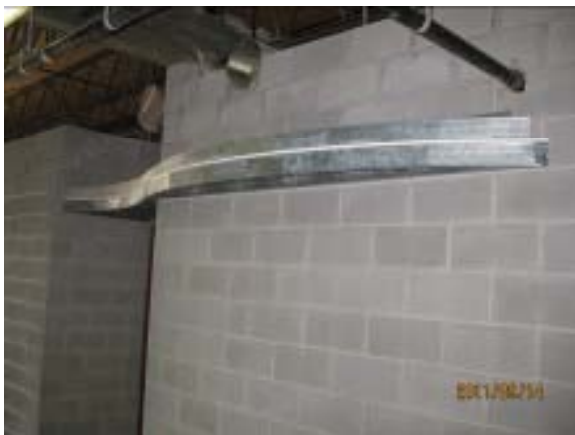
Soffit / Ceiling Construction
