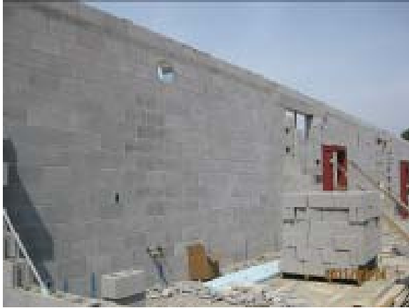
Masonry Walls – New Classroom Wing
