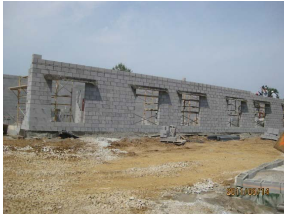
New Classroom Wing
