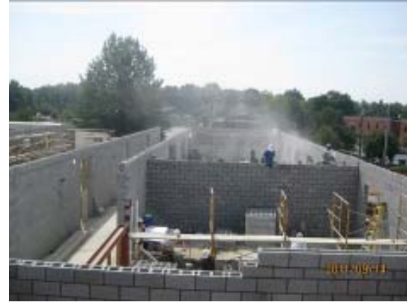
Top Out of New Masonry Walls
