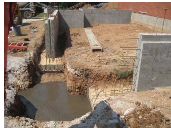
Stage Addition Foundation
