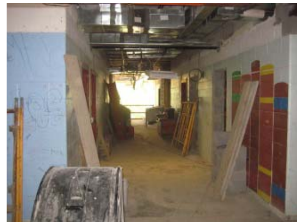
Corridor Demo Work
