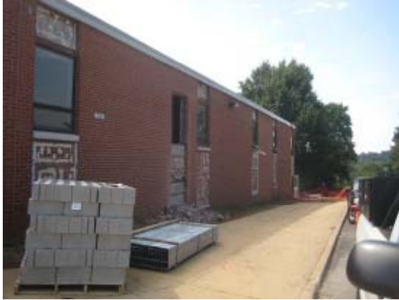
Front Elevation Demo Work
