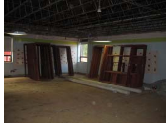
Lower Level Demo Work
