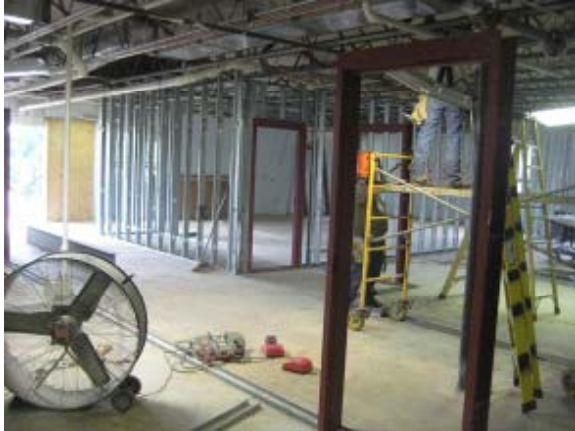
Metal Framing Installation
