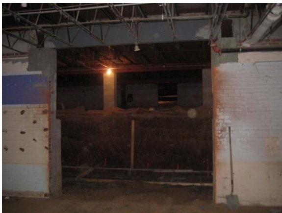
Lower Level Excavation
