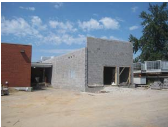
Mechanical Room Addition
