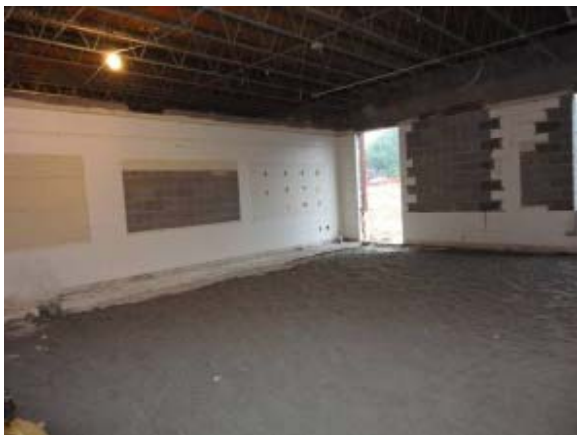
Pipe & Gravel Base New 1 st Fl. Slab
