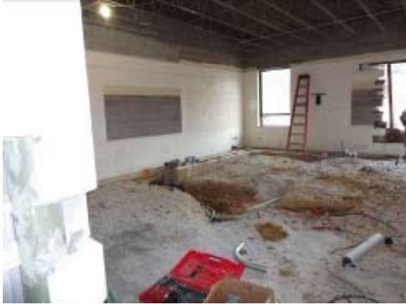
Underslab MEP Rough In
