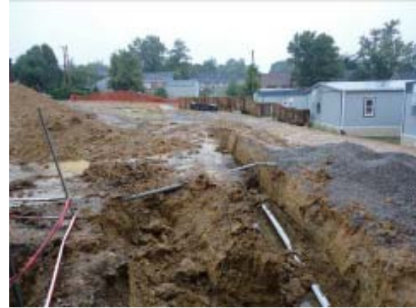
Trenching for New Utilities
