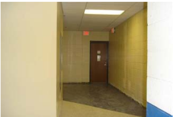
New Terrazzo Floors & Doors
