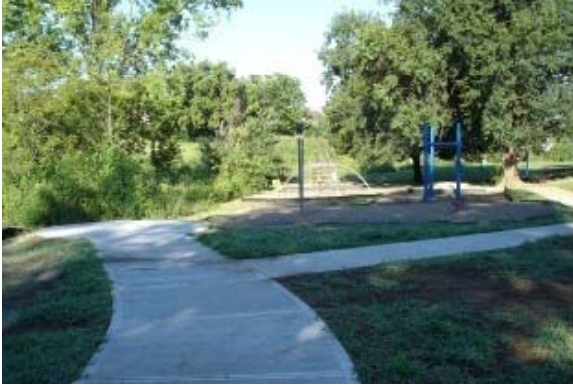
New Accessible Path to Stream & Playground
