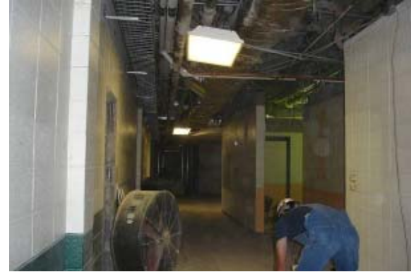
Renovation Inside Existing Bldg.
