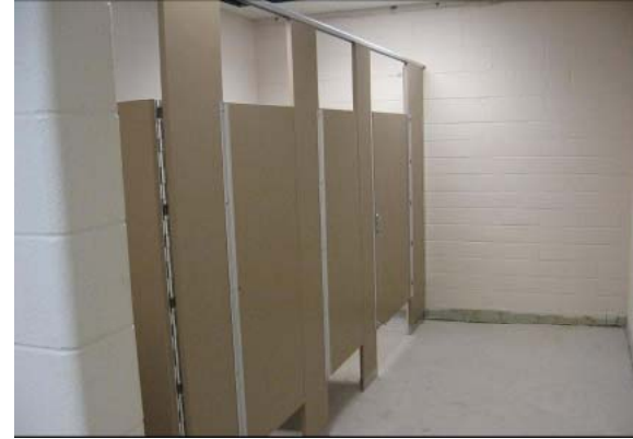
Phase Ia Bathroom
