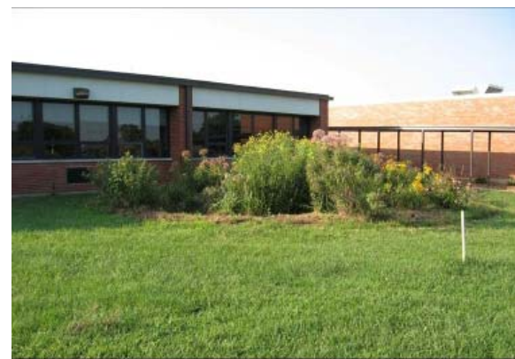
Existing Rain Garden
