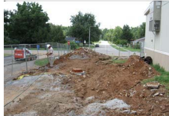
Site Utility Work
