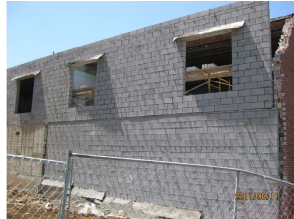
New Block Walls
