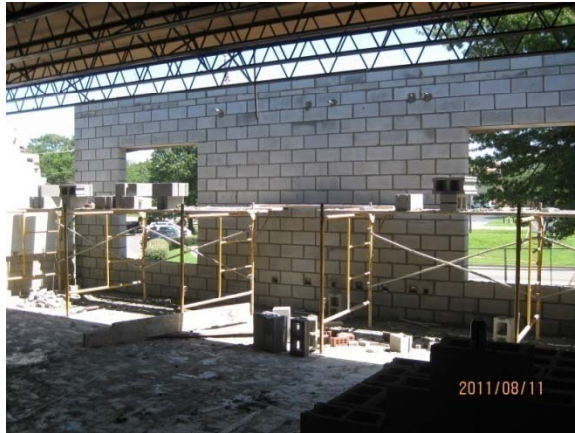
CMU Walls in Renovated Area
