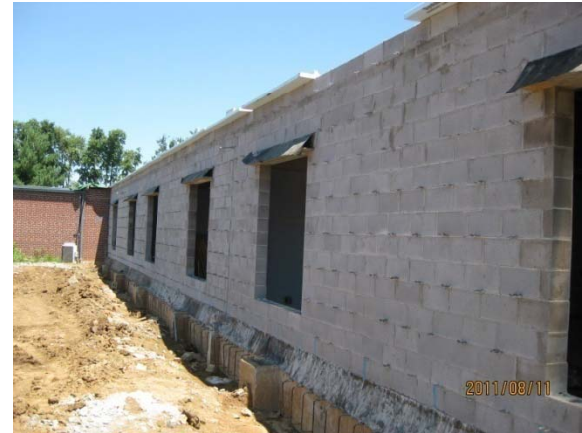
New Block Wall
