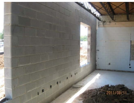
Interior New Block Wall
