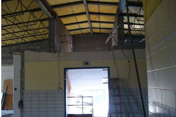
Upper Level Demo
