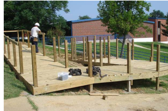
Temp Ramp to Cafeteria
