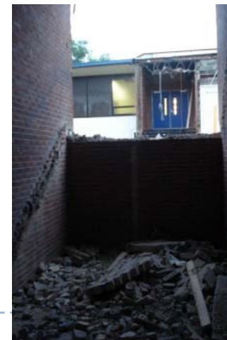
View from Lower Level Where Connector Removed
