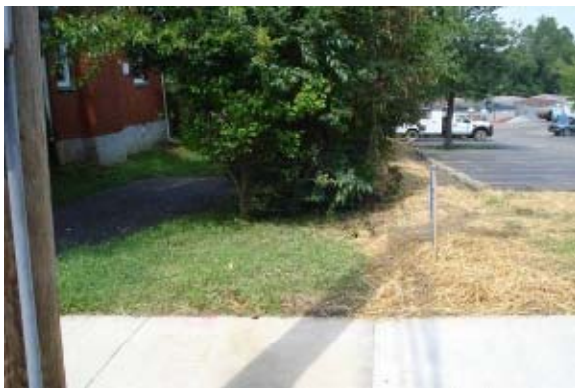
New Water Line Installed
