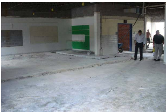
Interior Demo in 2-Story Classroom
