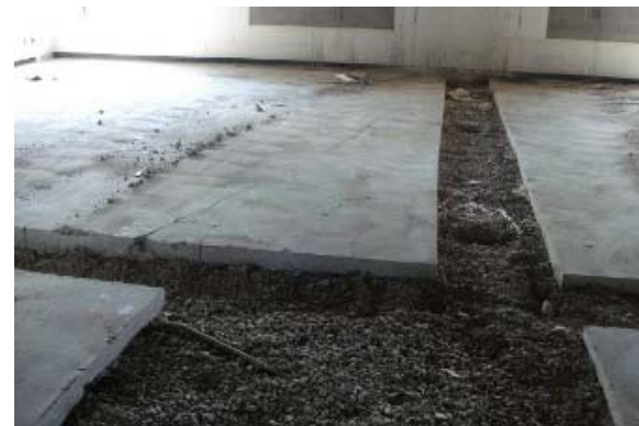
Trenching for New Utilities & Walls
