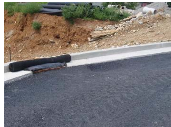
Asphalt Base Course
