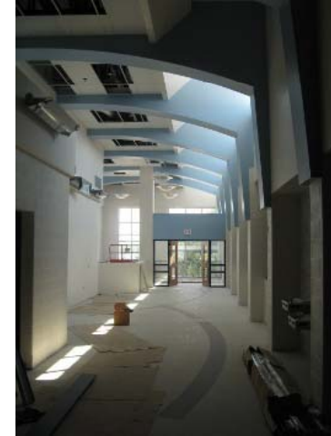
Ceiling Tile Near Complete
