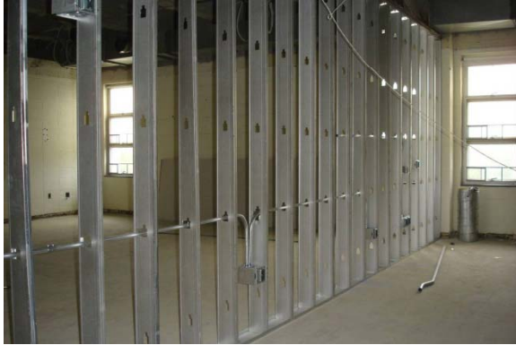
New Classroom Walls (replacing Operable Partitions)
