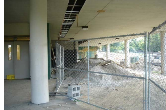
Electrical Room Installation
