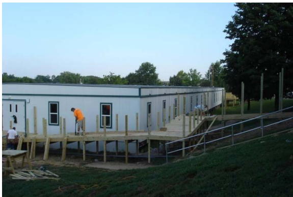
Multiplex Portable Classroom
