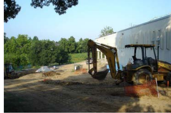
Re-grading Behind School for Access to Stream
