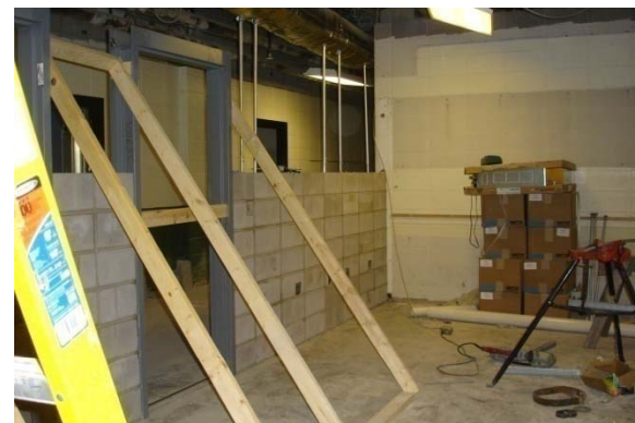
Doorframe Installation
