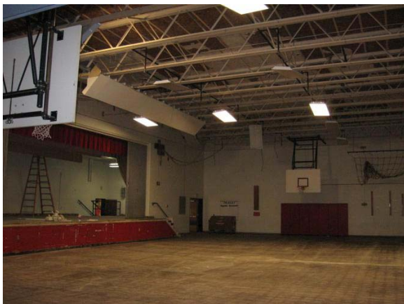
Gym – Abatement Work
