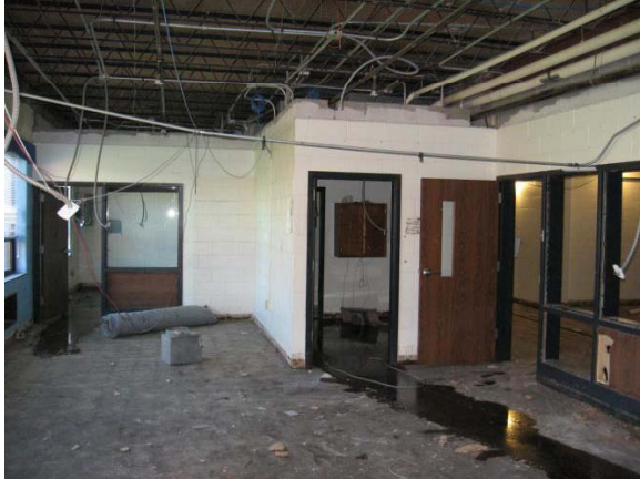
Admin Suite – Abatement Work
