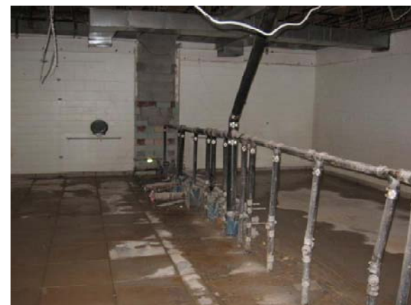
Bathroom – Demo Work
