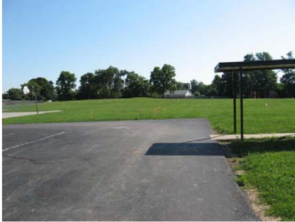
Site Staking for New Work
