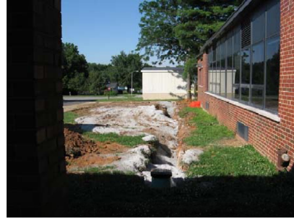
Site Utility Excavation
