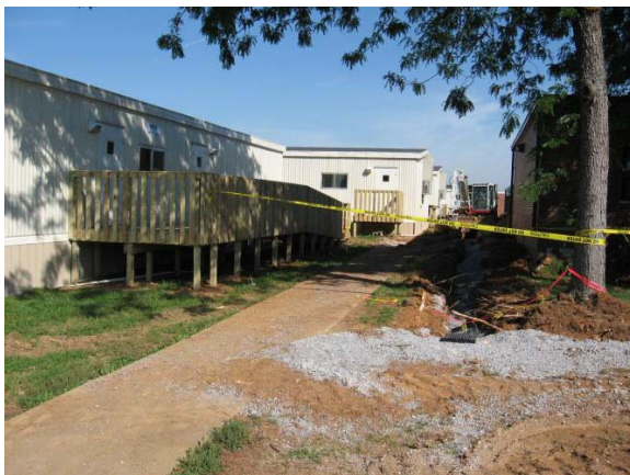
Utility Work for Portable Classrooms
