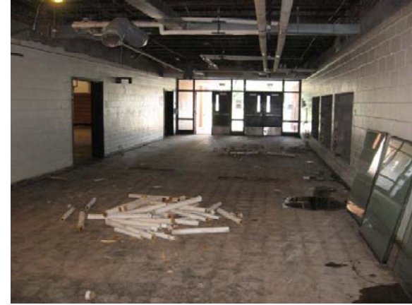
Lobby – Abatement Work
