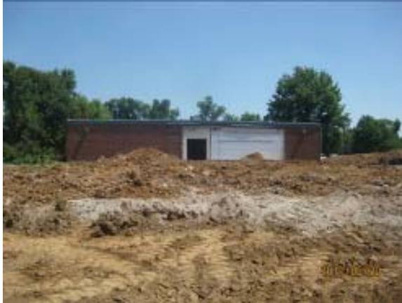
Demo for new Classroom Addition
